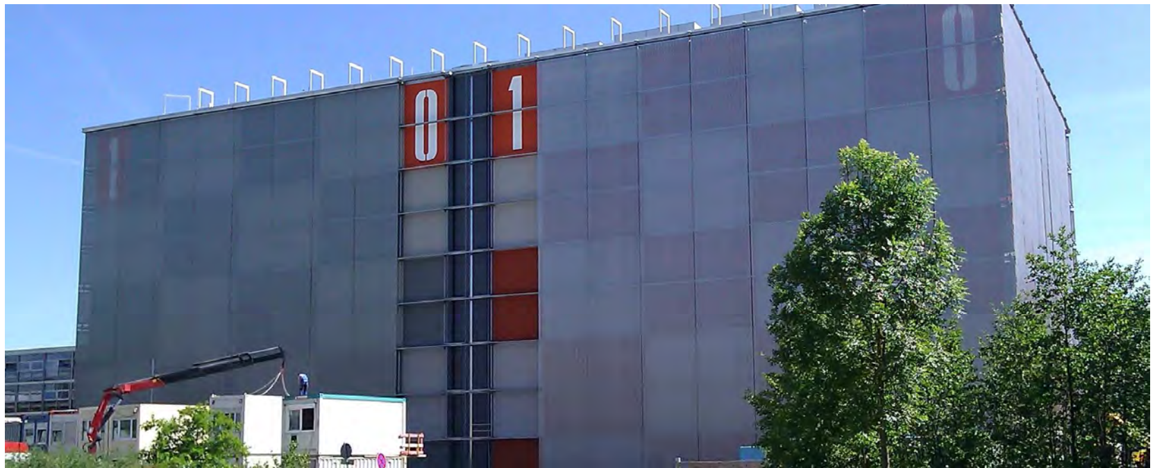
„Twin Cube“ with computing rooms (3,160m 2 for IT equipment, 6,393m 2 for Infrastructure, 2x10MW Power supply)
